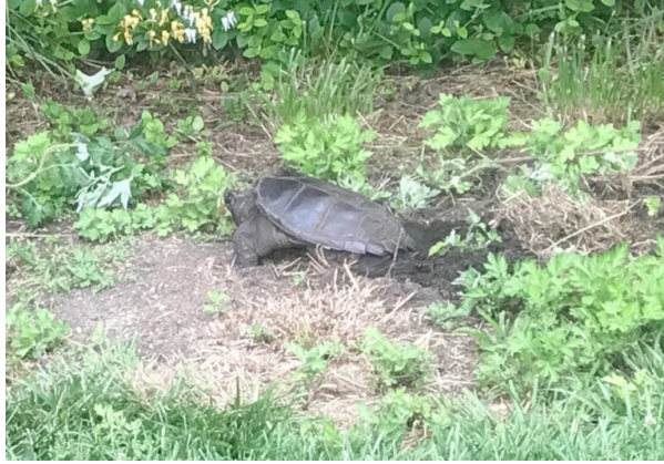
Bottom left, turtle peeks out from beneath his shell in Babylon Village as work on the Carlls River proceeds.
